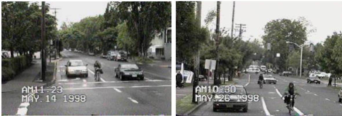
**Figure 37. Two configurations of combined bicycle lane/right-turn lanes**
