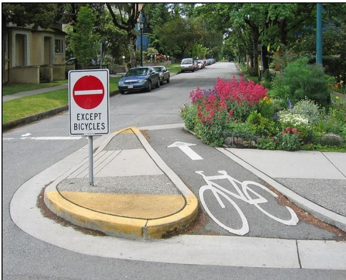
**Figure 42. Traffic calming that allows bicycle through travel while limiting through vehicle travel.**
