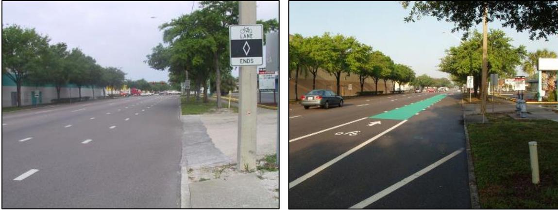
**Figure 40. Before and after photos of the installation of a green bike lane weaving area in St. Petersburg, Florida.**
