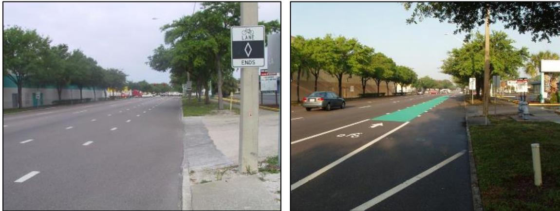
**Figure 14. Before and after photos of the installation of a green bike lane weaving area in St. Petersburg, Florida.**
