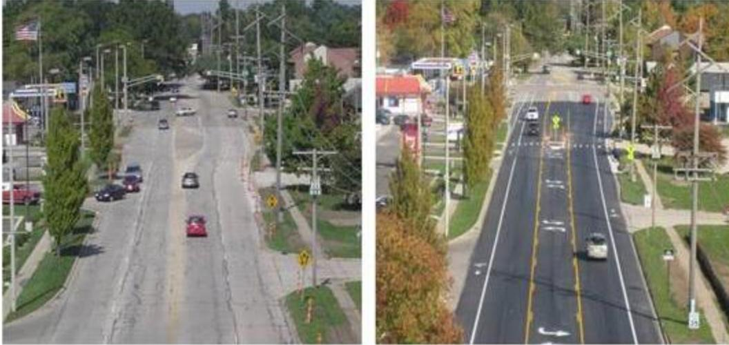
**Figure 3. Before and after pictures from Urbana, Illinois, illustrate a typical road diet project.**
